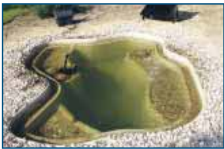
10. Filling and compensating In the final step the area around the preformed pond is adapted to the preformed pond with sand, soil, gravel, etc.
