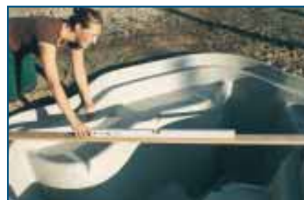
8. Levelling The preformed pond is inserted and levelled out in length and width. Then fill with water to approximately 1/3 of the total volume.
